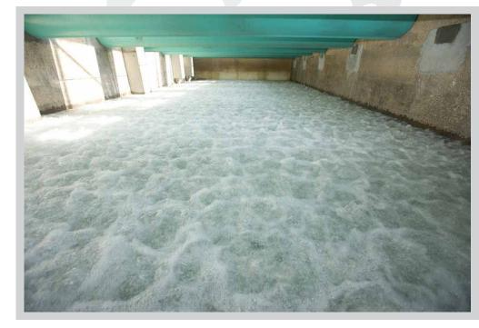
Typical air scour duration with The Phoenix<sup>™</sup> Air Scour System ranges from 3-5 minutes and may vary depending on site conditions, but can be as long as needed. Available in ranges from 2-10 cfm / ft² and beyond.
