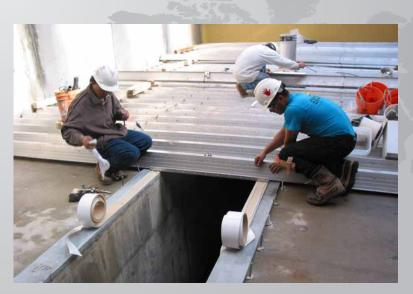
The Phoenix™ Underdrain is a complete system designed for all types of filters. Here is a typical gullet installation in a new filter with a 3 foot wide gullet. AWI is the only manufacturer that can accommodate a gullet width greater than 2 feet.
