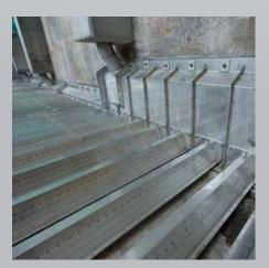
This filter retrofit feeds backwash water along the 50' wall. The custom designed feed box permitted the addition of more media than any other design, while distributing backwash water to the section of the feed wall that was not connected to the backwash supply.
