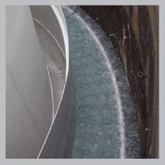
This is a custom retrofi of an Aldrich unit. The retrofit increased the depth of the filter media and added air scour. The available filtration area was
