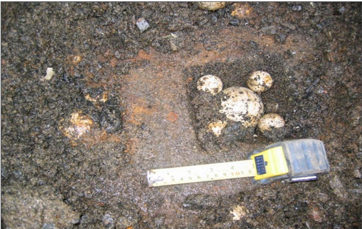
Existing Wheeler Bottom Underdrain
