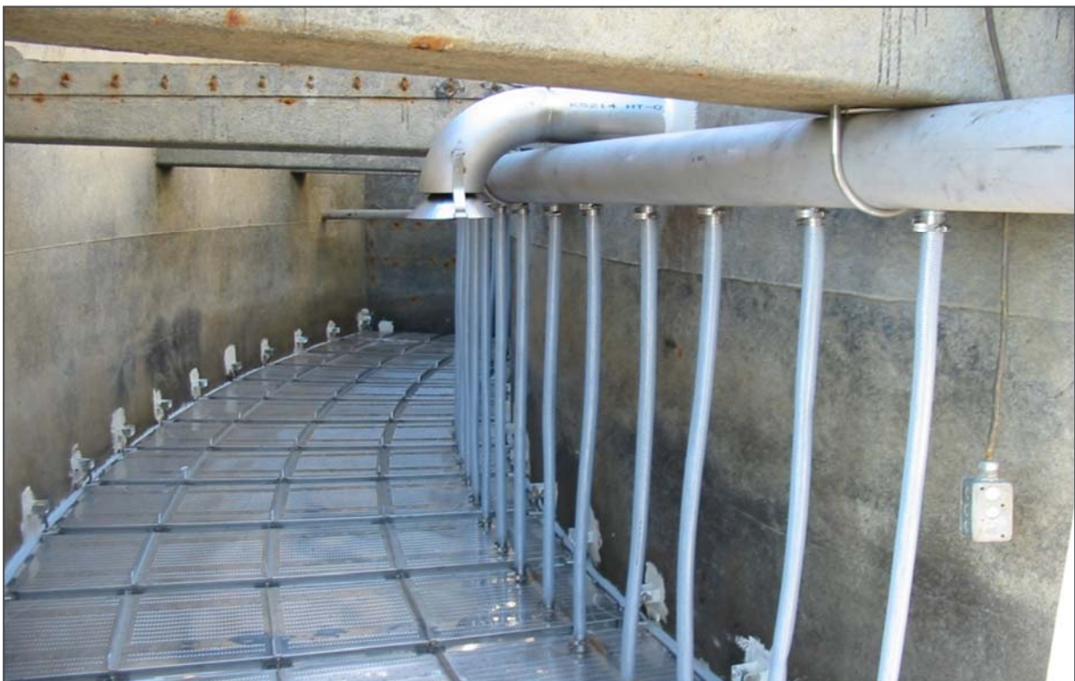
Air scour header connection to internal air conduit of Phoenix Panels
