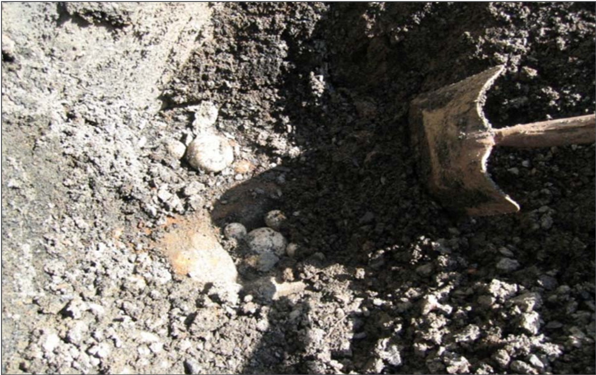
Existing Wheeler Bottom Underdrain
