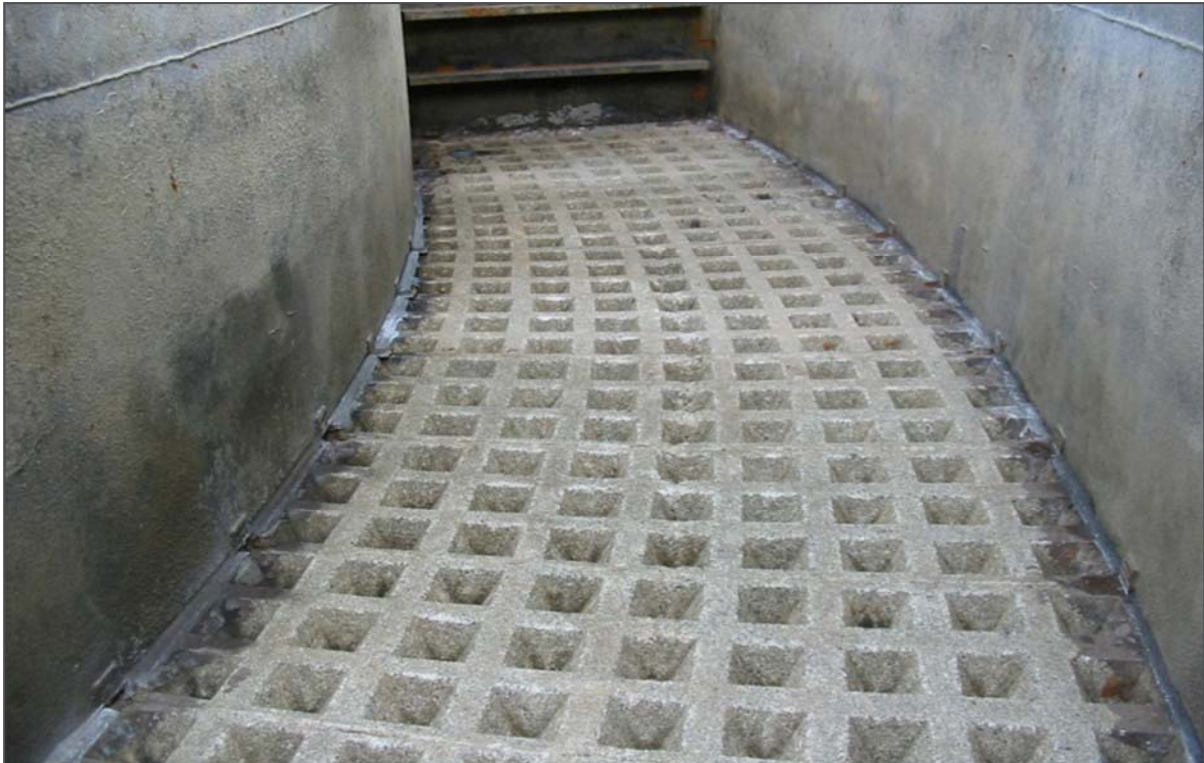
Filter and plenum prepared for Phoenix Panel installation
