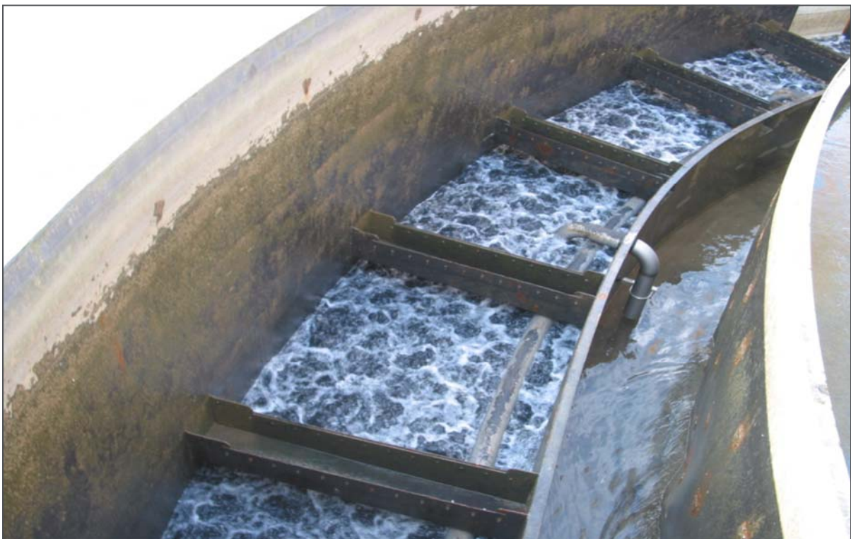
Air scour distribution testing
