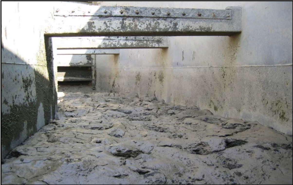
Condition of existing filter media bed
