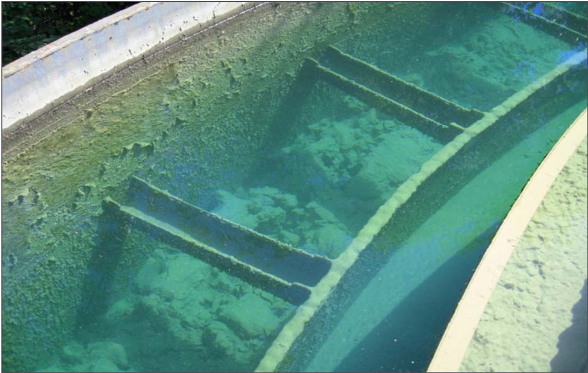
Condition of existing filter media bed
