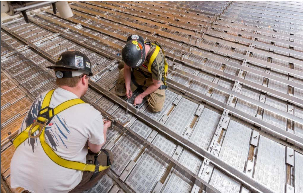
Installation of Phoenix Air Scour Grid
