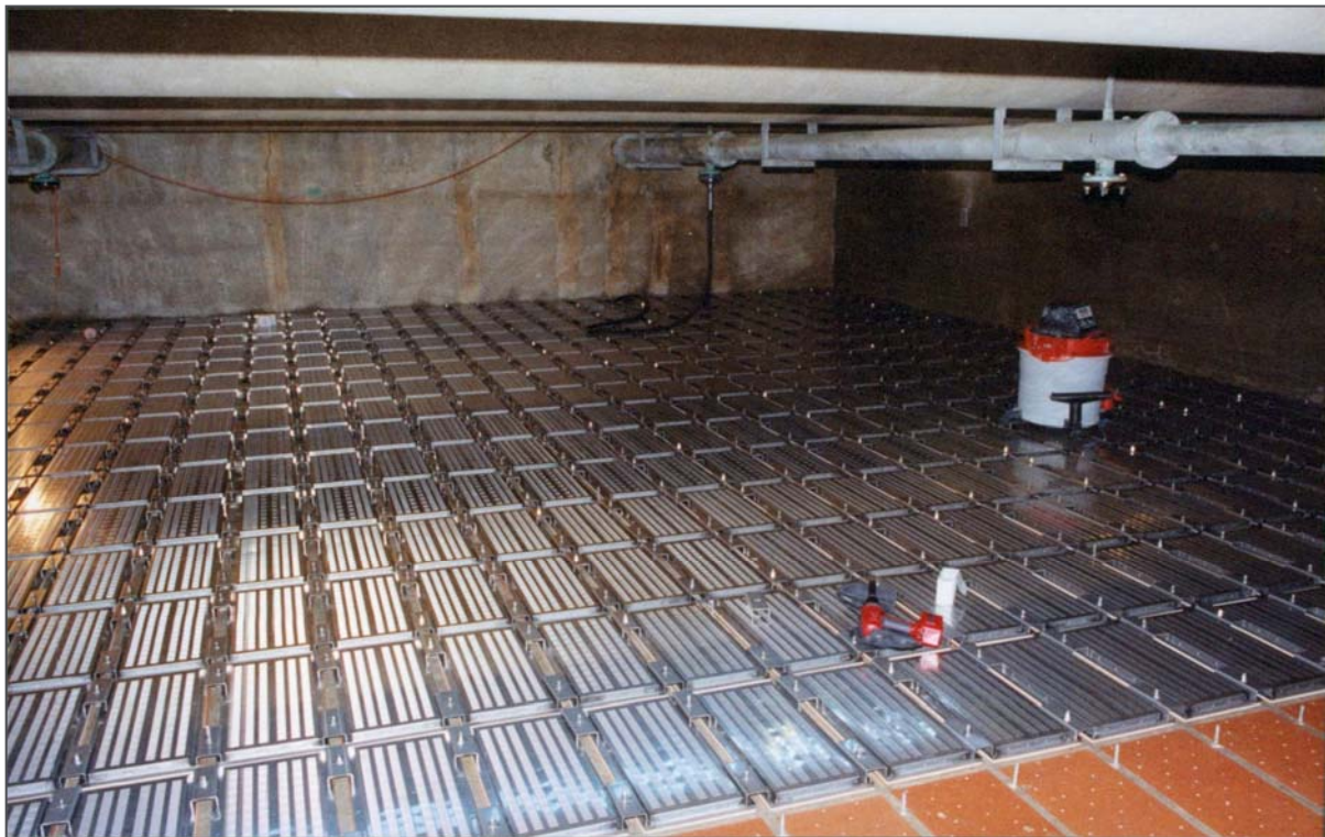
Installation of Phoenix Panel System
