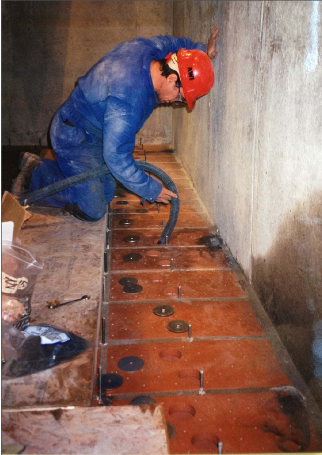
Coring and pressure washing of clay tile block to remove built-up debris
