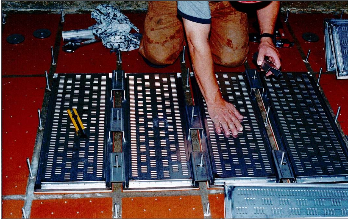
Installation of Phoenix Panel System
