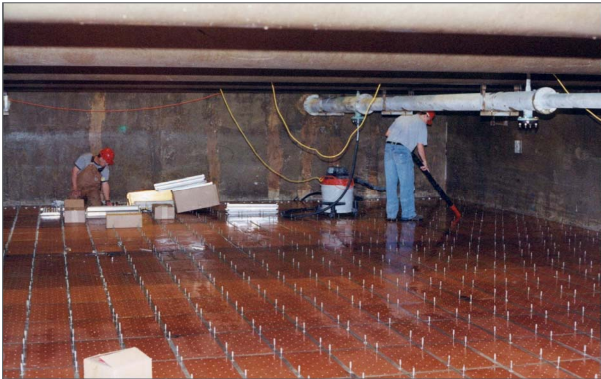
Preparation of filter floor for Phoenix Panel System installation
