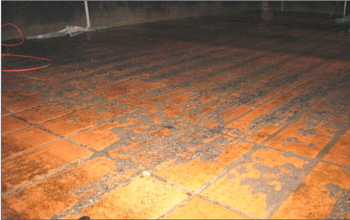
Existing clay tile block underdrain
