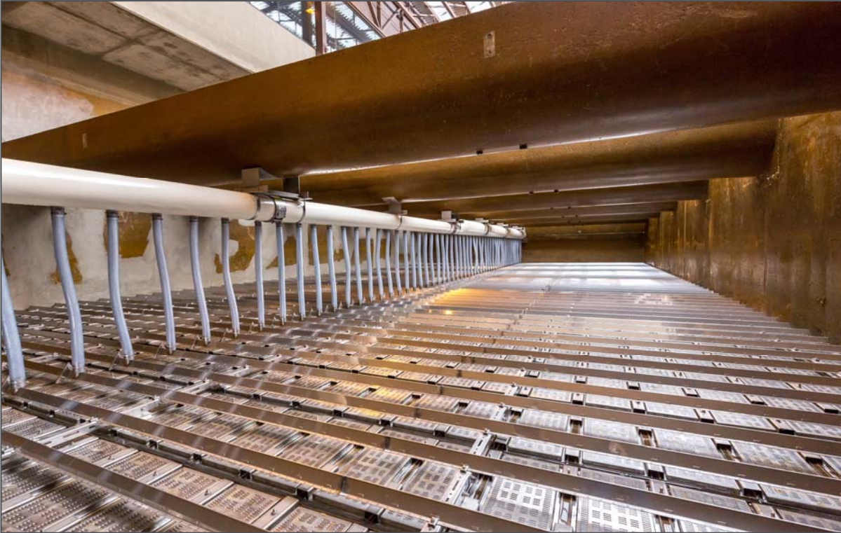
Completed Installation of Phoenix Air Grid
